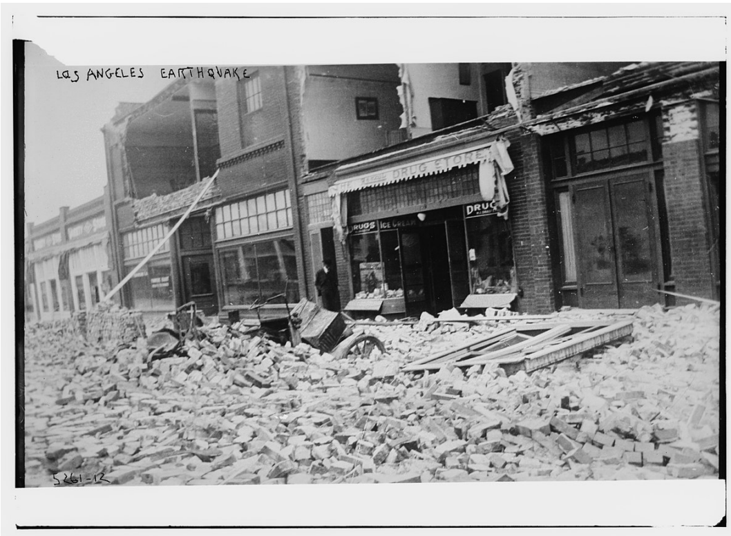
Aftermath of Los Angeles Earthquake (1920).
