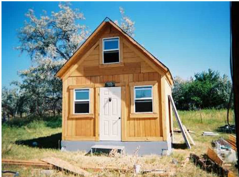
Here you can see how I finished the foundation. I used 5/8 wafer board painted grey to look like cement. Eventually I will rock the foundation with river stones. My trim work is all rough cut pine 1x6s I get directly from a small lumber mill up the road.
