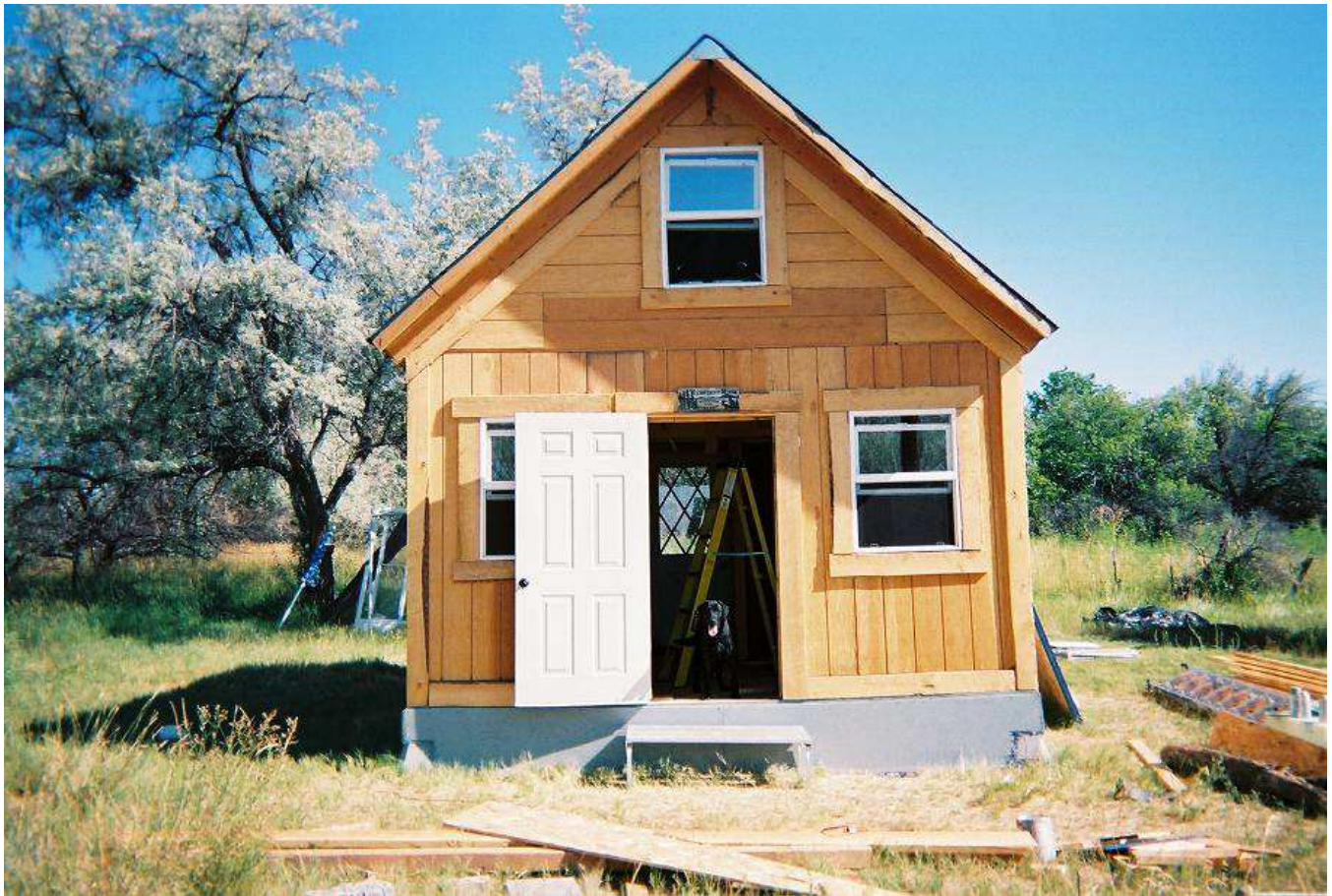
Front of cabin under construction
